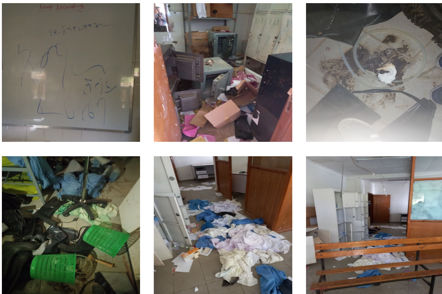
Figure 13: Photographs showing the destruction of Ataye Hospital.
