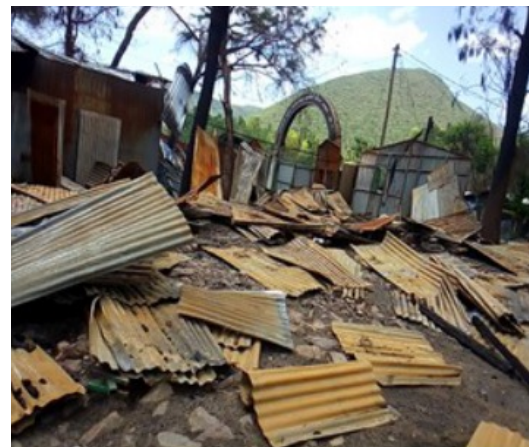
Post-attack situation of Woreda Administration Offices 1/2
