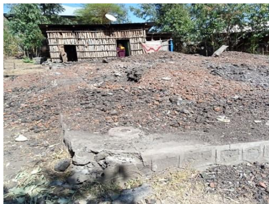
A residential house that was deliberately burned down by the TPLF militia
