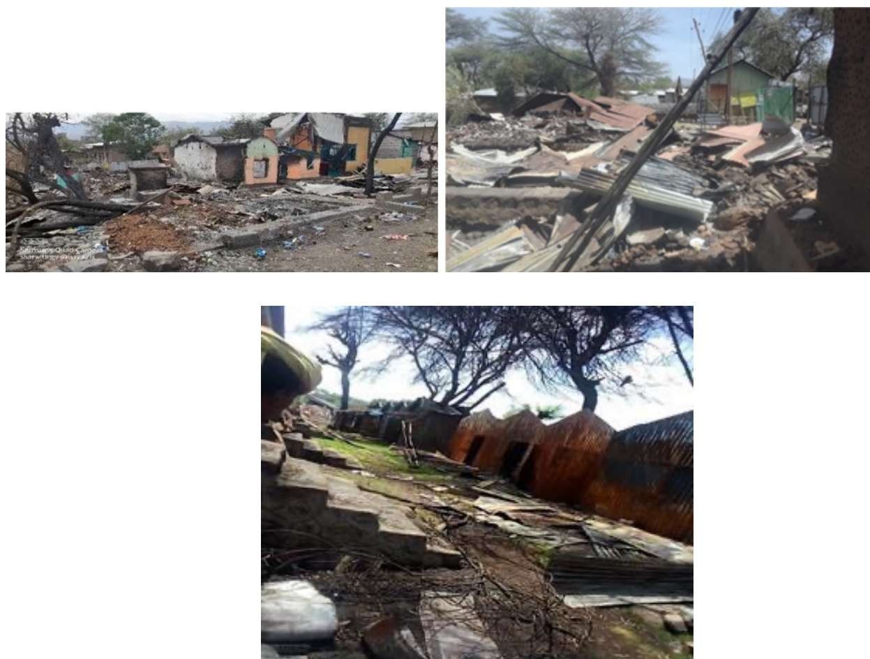
Figure 7: Roadside-facing buildings were looted first and set ablaze in Ataye town.
