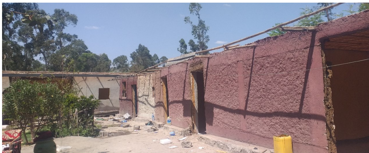
Yimam's house under demolition
